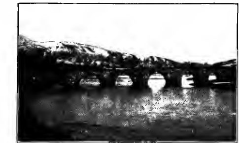
FIG. 11.—Roman Bridge over the Halys.
